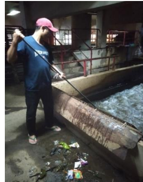
Gambar 3.5 pembersihan bak screening
