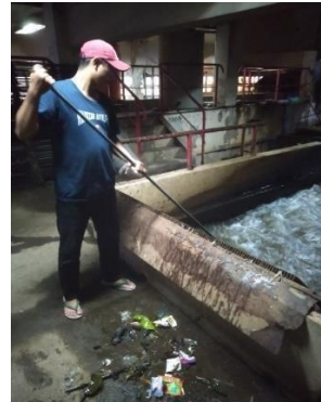
Gambar 3.5 pembersihan bak screening
