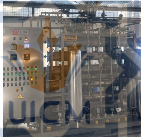
Gambar 4. 7 Sistem Reverse Osmosis (RO)
