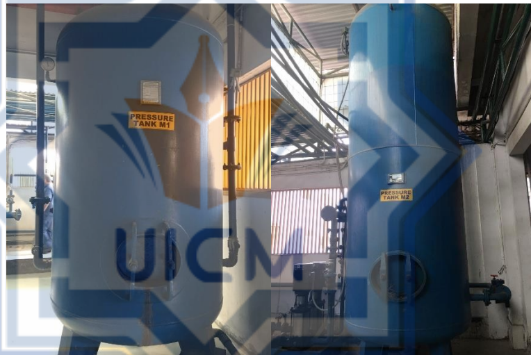
Gambar 4. 4 Pressure Tank Mepro-1 dan Mepro-2
