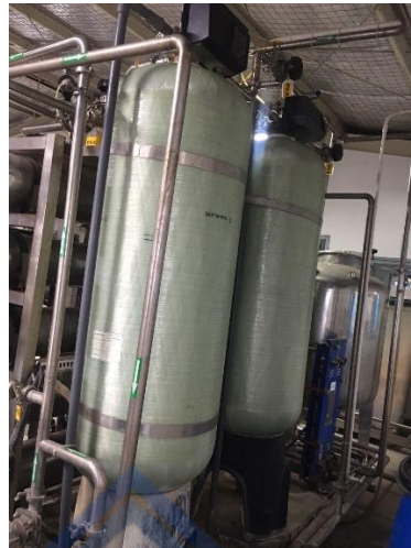
Gambar 4. 6 Softener Resin kation
