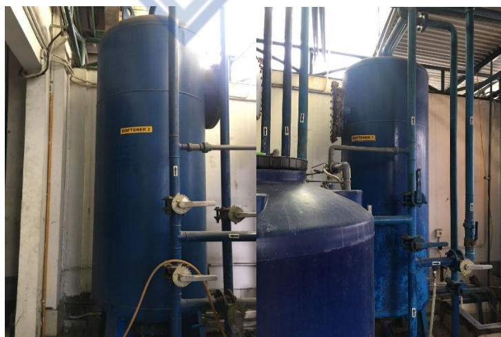
Gambar 4. 5 Softener Tank 1 dan 2
