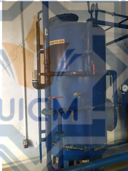
Gambar 4. 2 Sand Filter
